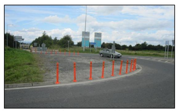
Figure 16: Example of a temporary stone road on central island of roundabout
