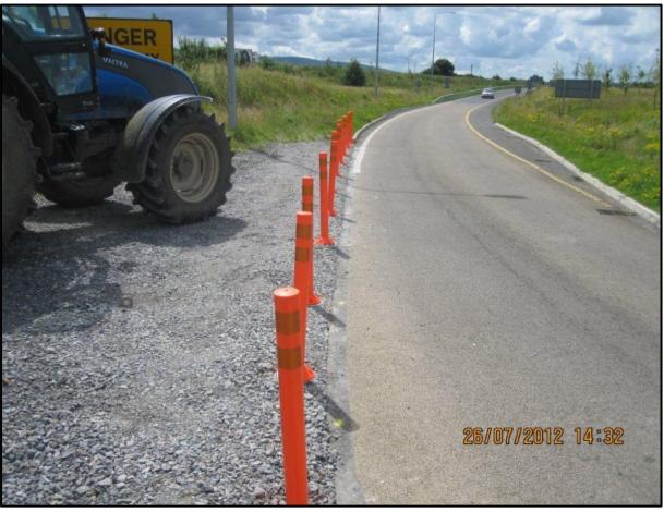
Figure 22: Example of temporary road widening along an off-ramp.
